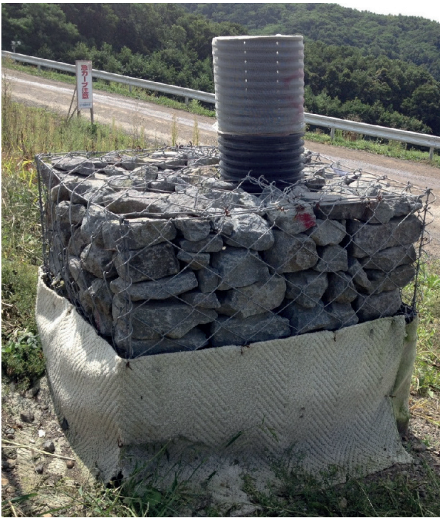
FIGURE 2: A typical landfill gas venting pipe.
