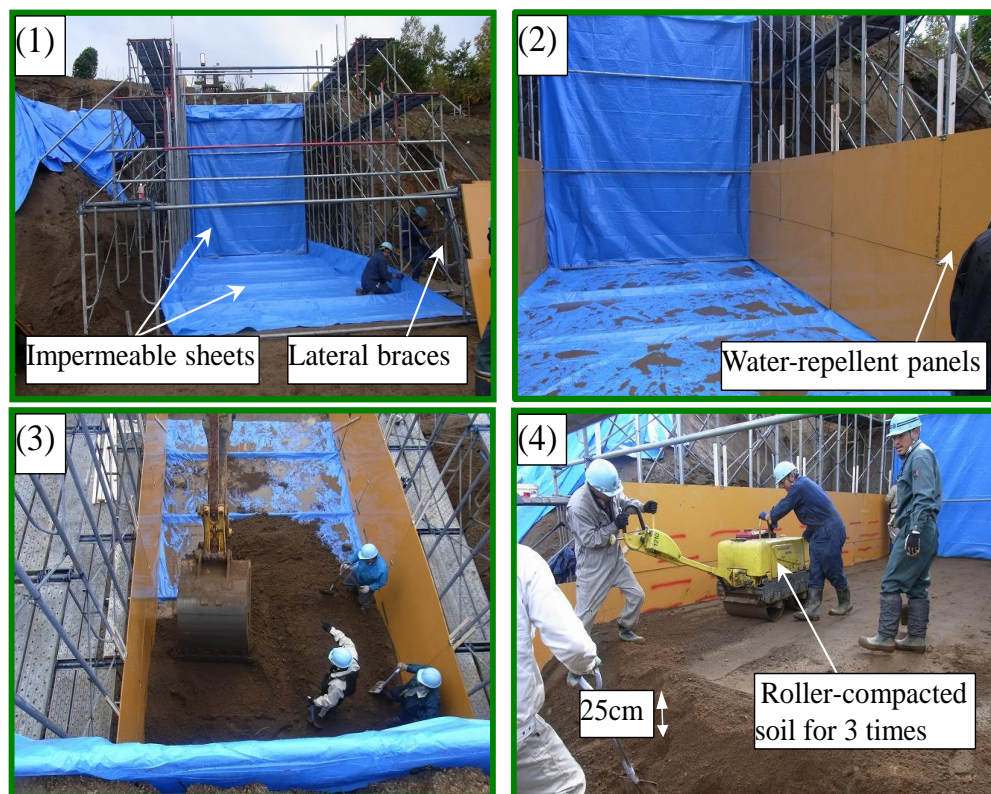
Figure.2.23 Construction procedures of FE-1212: (1) setting impermeable sheets and lateral braces; (2) setting water-repellent panels; (3) Filling soil; (4) Compacted soil
