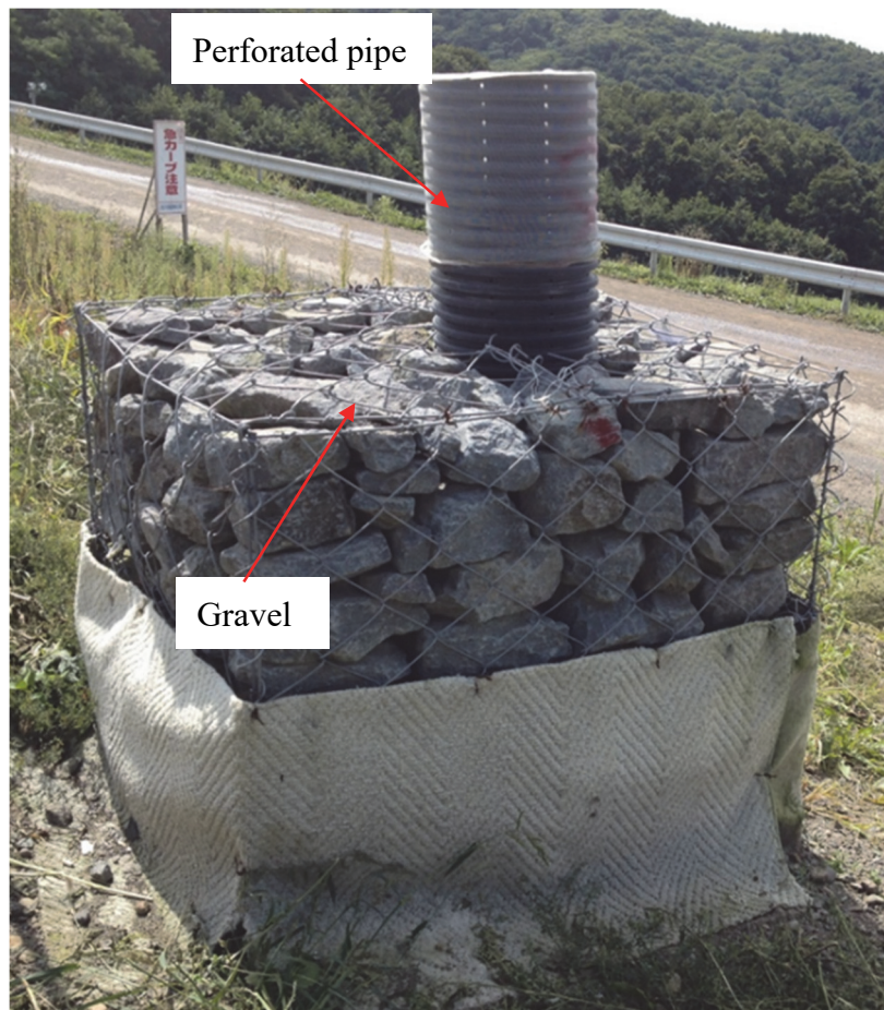
Figure 3 A typical landfill gas venting pipe (venting pipe)
