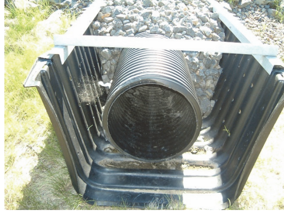
Figure 11 Main leachate collection pipe (perforated pipe)
