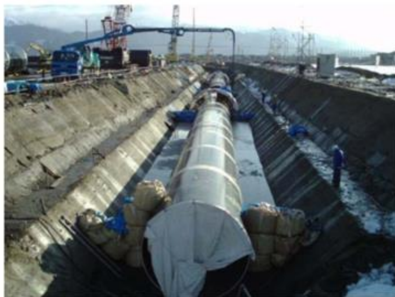
Figure 2.12 Backfilling of LSS
