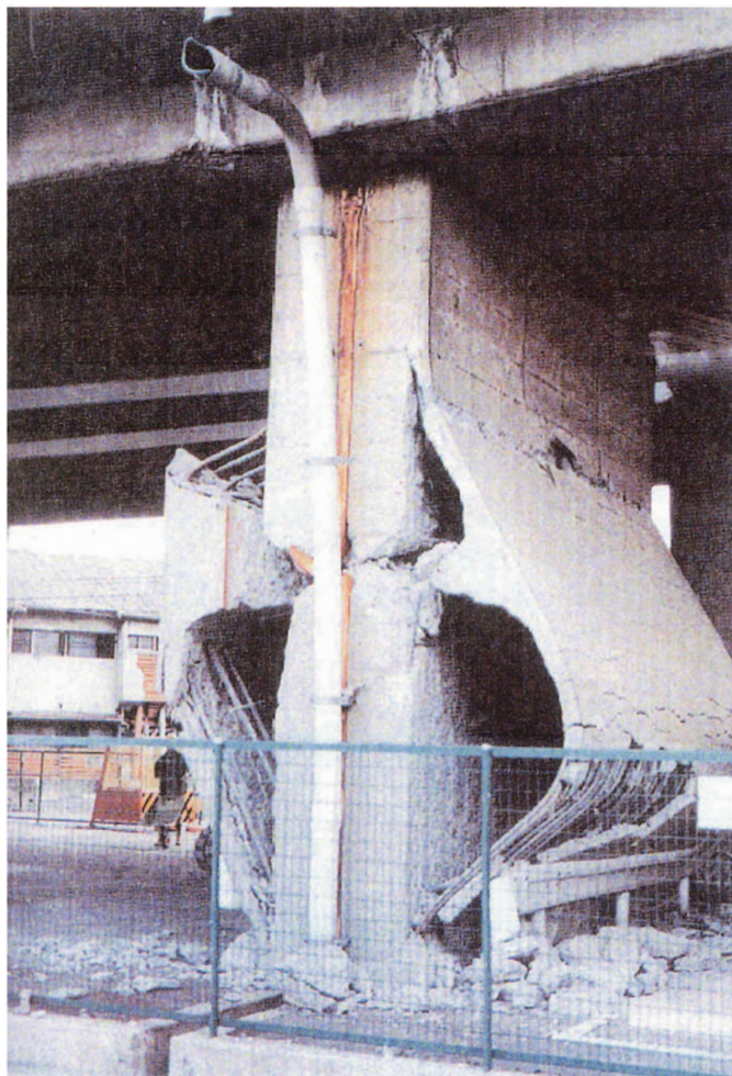
Fig. 1. (Color) Example of the compression failure of an RC bridge pier. (Image by Keiichiro Sonoda.)
