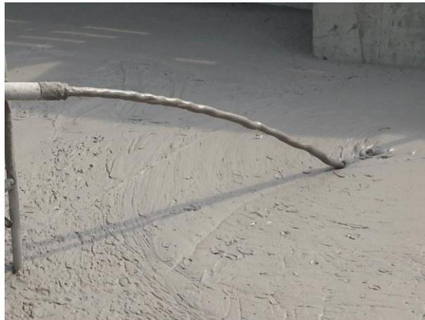
**Fig. 1.6** Lightweight air-mixed soil
