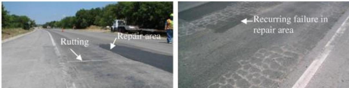
**Fig. 1.3** Recurring failure in repair area (Chen et al., 2013)
