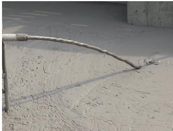
Fig. 1.6 Lightweight air-mixed soil
