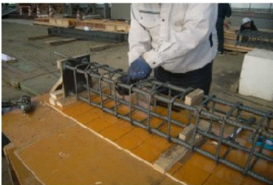
(a) Formwork and reinforcement
