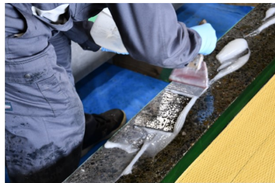
(b) Epoxy resin application
