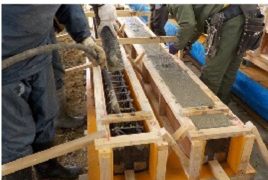
(b) Concrete casting
