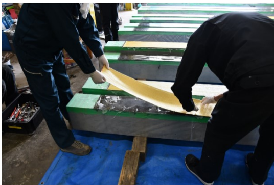
(c) AFRP sheet bonding
