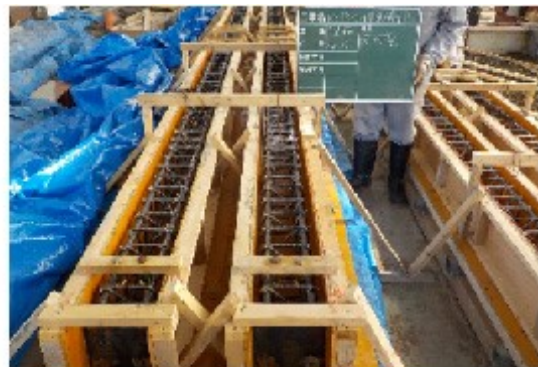
(a) Formwork and reinforcement
