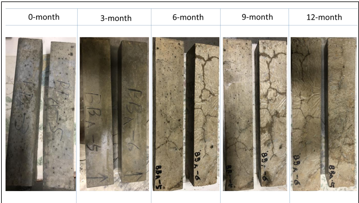
Fig. 5-3 cracks in AB-N due to ASR
