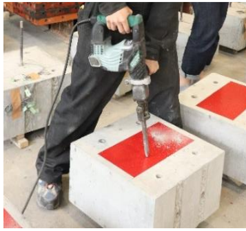
(a) Roughening by a hammer
