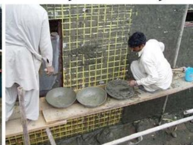
Figure 2.2. PP band mesh retrofitting procedure for masonry house
