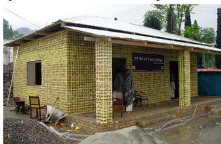
Figure 2.2. PP band mesh retrofitting procedure for masonry house
