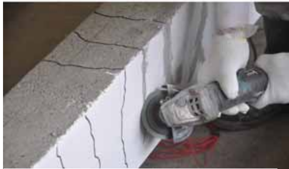
(a) Preparing the cracks surfaces
