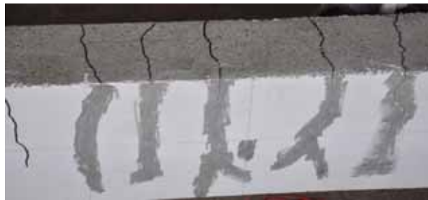
(a) After preparing the cracks surfaces
