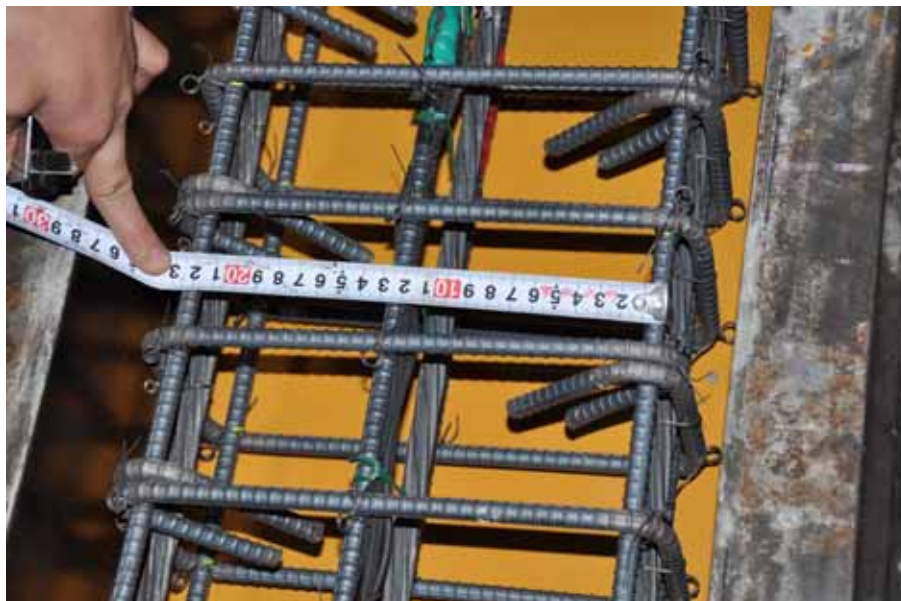
(b) Rebar steel
