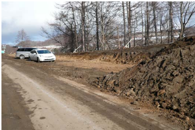
Photo 7.3 Construction site at Route “Abuta - Toya”, Hokkaido Pref. Highway
