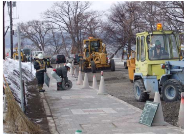
Photo 7.2 Construction site at Route "Lake Toya - Noboribetsu", Hokkaido Pref. Highway
