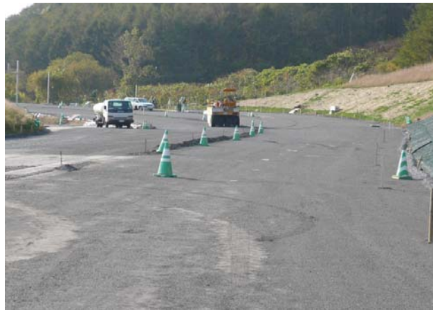
Photo 7.1 Construction site at Abuta-Lake Toya IC, HOKKAIDO EXPWY
