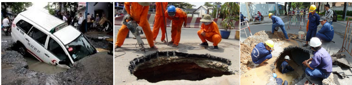
Figure 2.13 Cave-ins and road collapses in Ho Chi Minh city
