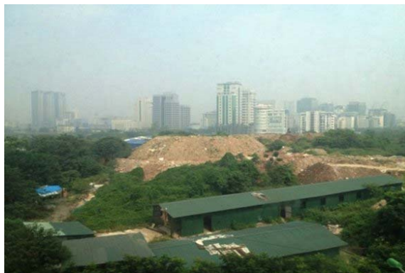
Figure 2.11 inappropriate disposal of excavated soils from construction sites in Hanoi
